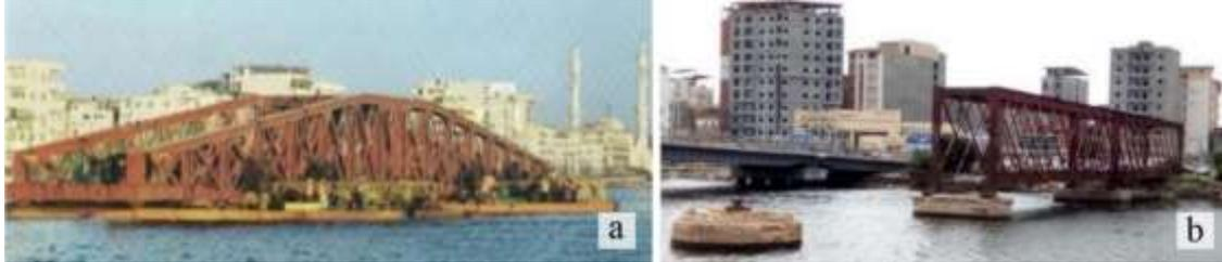
Fig. 4. a. The Movable Segment of Damietta Bridge during the Relocation [28]; b. The Remaining Fixed Parts of Damietta Bridge, photo by S. Sheweka.
