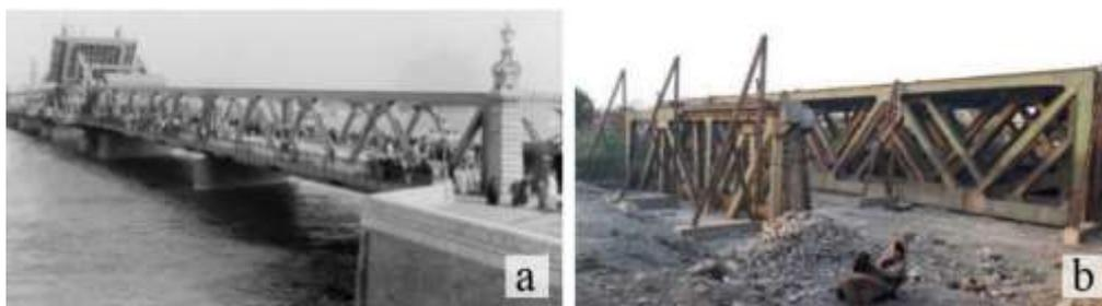
Fig. 3. a. Boulaq Bridge before Dismantling, b. Boulaq Brige after Dismantling, Author's Collection.
