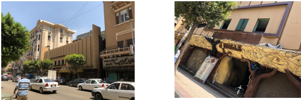
Fig. 7. Cinema Elkahira before and after painting with the removal of the name protruded on the vertical tower.
