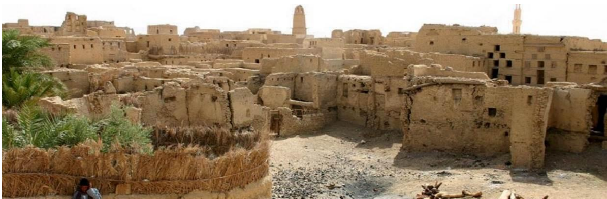
Fig. 18. A part of the old city suffers from neglect, cracking and demolition.
