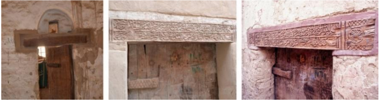
Fig. 9. The wooden sills above the doors with the house construction year [12].
