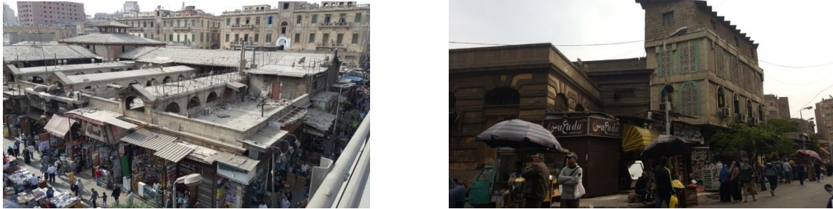
Fig. 10. Second skin of shops covering the market facades, a multi-story building covering the façade of Mohamed Ali street.
