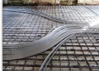
Electrical and mechanical network installations.
