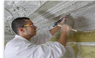
Tiny cracks curing.
