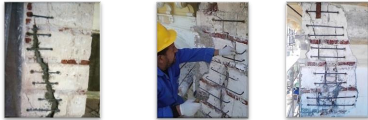
Tearing façade cracks process and installation.
