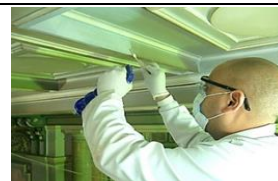
Mechanical and chemical cleaning for internal ceilings.
