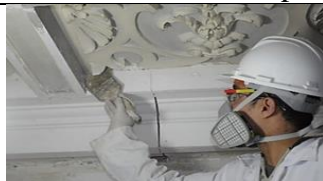
Mechanical and chemical cleaning for internal ceilings.
