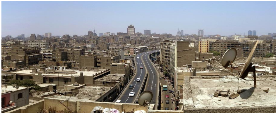
Fig. 8. The flyover contrast within its surrounding, Google Earth.
