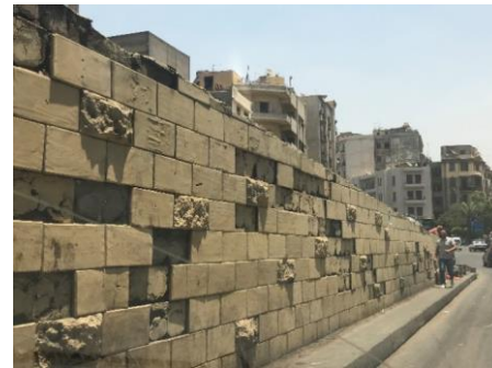
Fig. 4. Flyover abutment clad with bricks.
