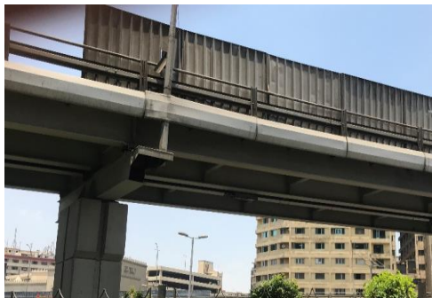
Fig. 3. Flyover barrier and railing.
