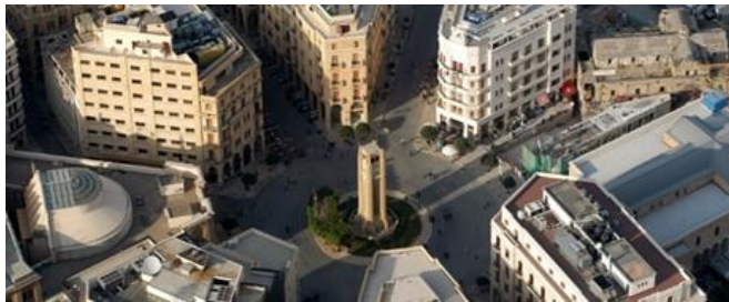
Fig. 1. Beirut city center after reconstruction [25].
