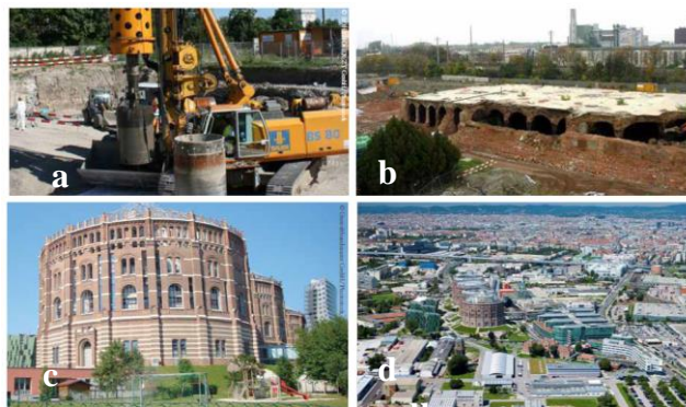
Fig. 5. a. Large diameter boreholes and steel piling coffer, b. The elimination of tar storage, c. Gasometer city, d. Aerial view operations center of “Wiener Netze” [31].
