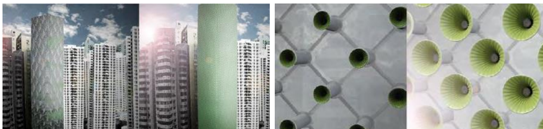
Fig. 9. Membranes used in the envelope of the building to carry water, air and light [22].
