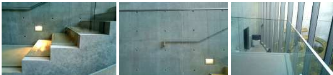
Figs. 27-29. Interior shots represent fairface concrete and non-mullion glass handrails. Photographed by the author, during visiting Tokyo, 2013.
